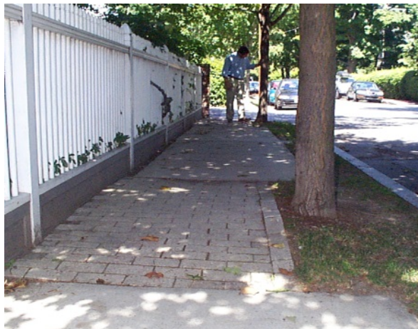
Figure 7: Sidewalk narrowed and pavers installed to provide more room for root growth
