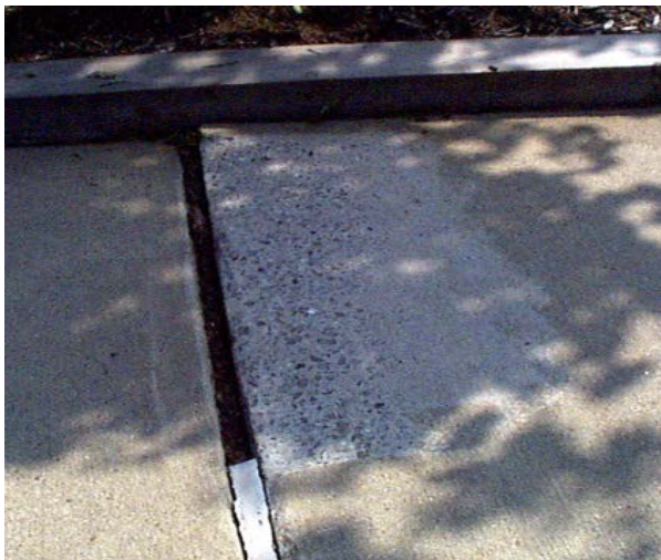
Figure 4: Asphalt ramp/wedge installed to reduce tripping hazard
