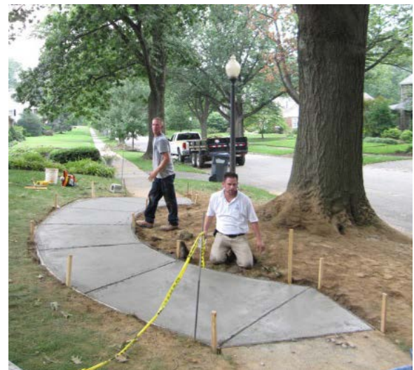
Figure 5: Sidewalk rerouted to increase the distance from the trunk and avoid root damage
