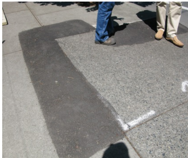
Figure 4: Asphalt ramp/wedge installed to reduce tripping hazard
