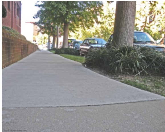
Figure 9: This new smooth and level sidewalk required root cutting within 1.5 times trunk diameter.
